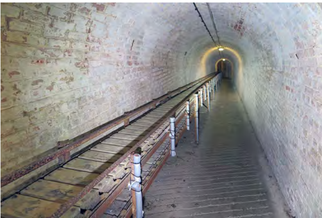
Ammunition conveyer leading down into the tunnels at Fort Nelson.
